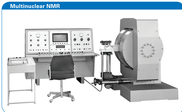
1967: HFX 90, the first fully transistorized NMR system, equipped with three independent channels.
