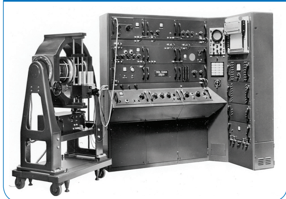
1960: 25 MHz permanent magnet KIS NMR system.
